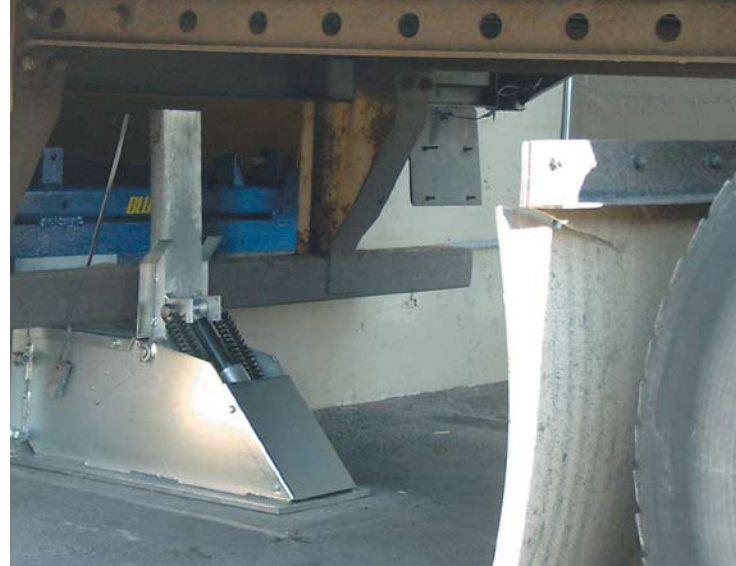
Look for ICC bar restraints that can confine a wide variety of bars—including bent bars—such as this one, which is a non-impact, swing-up arm.
